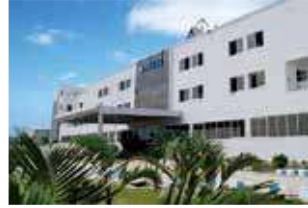
Rudrapur Plant (Green Building)
